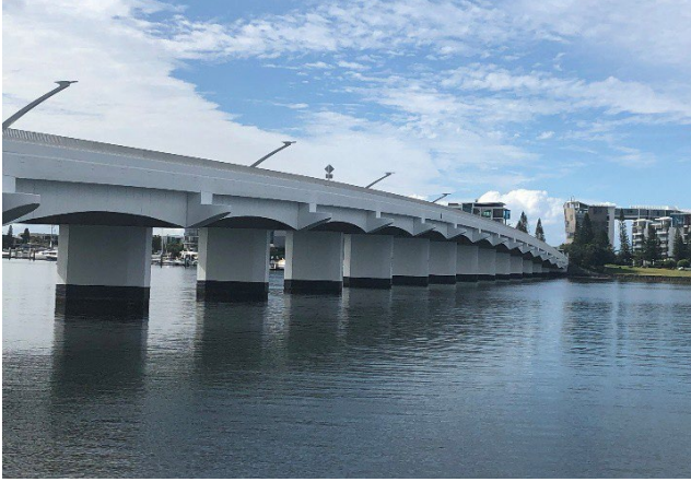
Barriers and Piers
